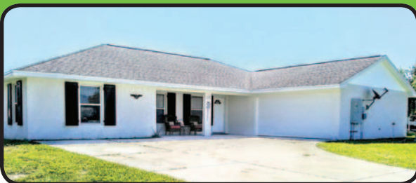
M-1846 Buckhead Ridge Beauty 3bd/3ba CBS home with a bonus room with its own entrance, great for guests, family, or an office, also has a 2 car garage and a screened in back patio overlooking the water on a captive lake. Immaculate and very well kept. Concrete slab for boat storage or trailers as well as a concrete drive and 2 sheds for storage. priced at $ 239,900. Call Theresa Kerr at 863-484-4769 for an appointment.
